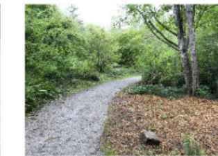
compacted gravel path
