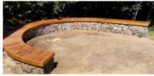
wood-topped gabion baskets
